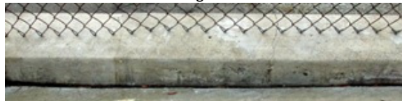
Concrete Curb After Cleaning with SB 2301
